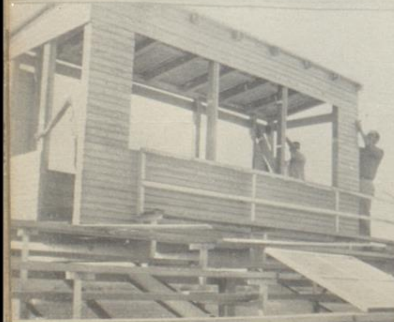
Ground Observation Station under construction.
