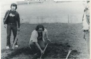
Ermino Arroyos shapes up the foundation as Cuevas and Gonzales check out the guide lines prior to pouring concrete. As part of the construction trades class instructed by Mr. Pittman, the students are learning how to set up an area for concrete foundations which will form the setting for the new oak trees to be planted in the area.
